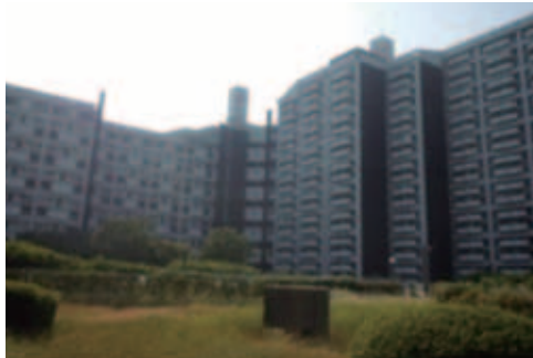
The surrounded central roof area converted to a green strip above the central shop (Photo courtesy of Norioki Ishimaru)
