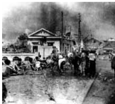
Photo taken at the Miyuki Bridge, immediately after the bombing (just past 11 a.m. on August 6, 1945). (Photo by Yoshito Matsushige, Courtesy of the Chugoku Shimibun)
